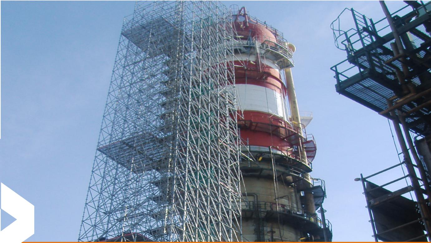
**Repsol Refinery in Spain.** *The assembly of the 90 metres high RINGSCAFF scaffold for sandblasting work at the refinery in Tarragona was a real statical challenge. The difficulties posed by the temperature fluctuations of the refinery, the increased wind load added by the protective tarpaulins, and the accumulating blasting material were solved with careful planning of the anchoring, a special configuration and perforated steel planks.*
