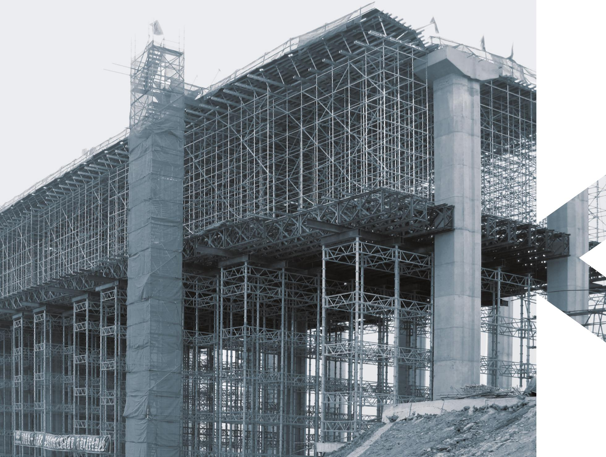
**Guilong Highway in China.** One million cubic metres of SPS, Duralok and SBS 135 material were used for the construction of the 12 km long Highway in the Guizhou Province. Special designs of shoring had to be done for the project.
