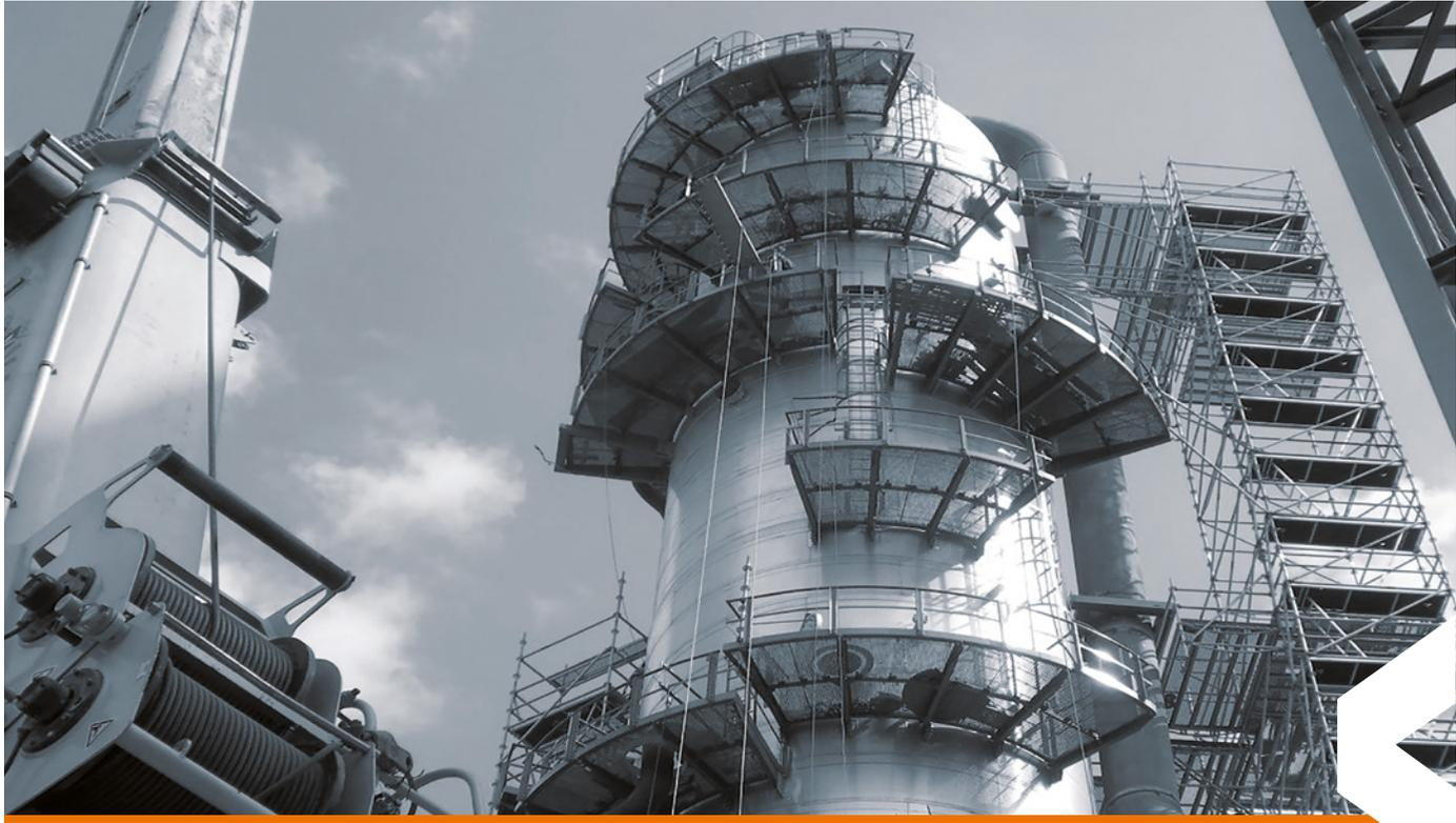
**Europoort Power Plant in the Netherlands.** *The multidirectional RINGSKAFF system was ideal for the work on the power plant in Rotterdam. Thanks to its flexibility, the scaffolding could be adapted to the challenging shape of the object.*
